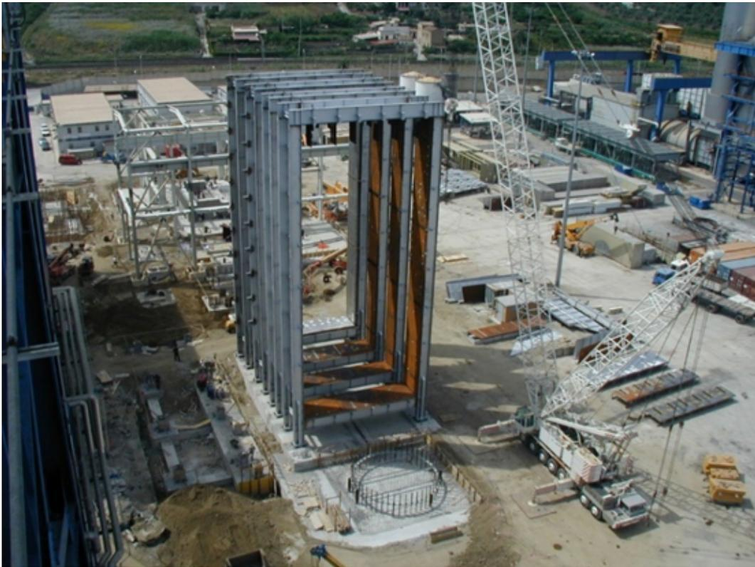
**Fig. 4 – Structural works – Steam generator Casing**
